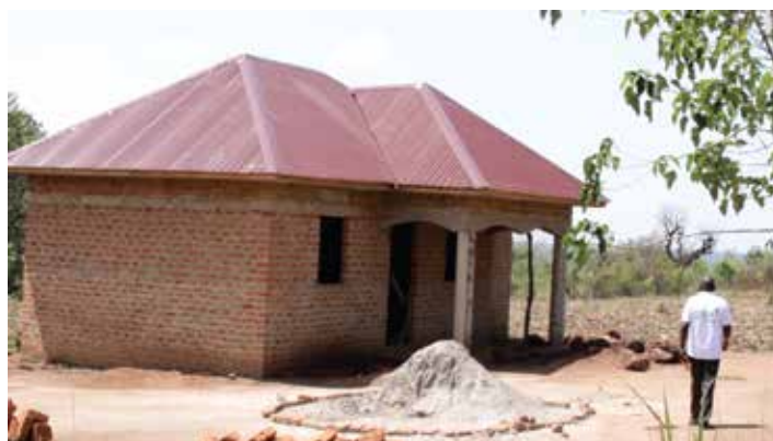
The side view of Omara Emmy's new house in-development.
